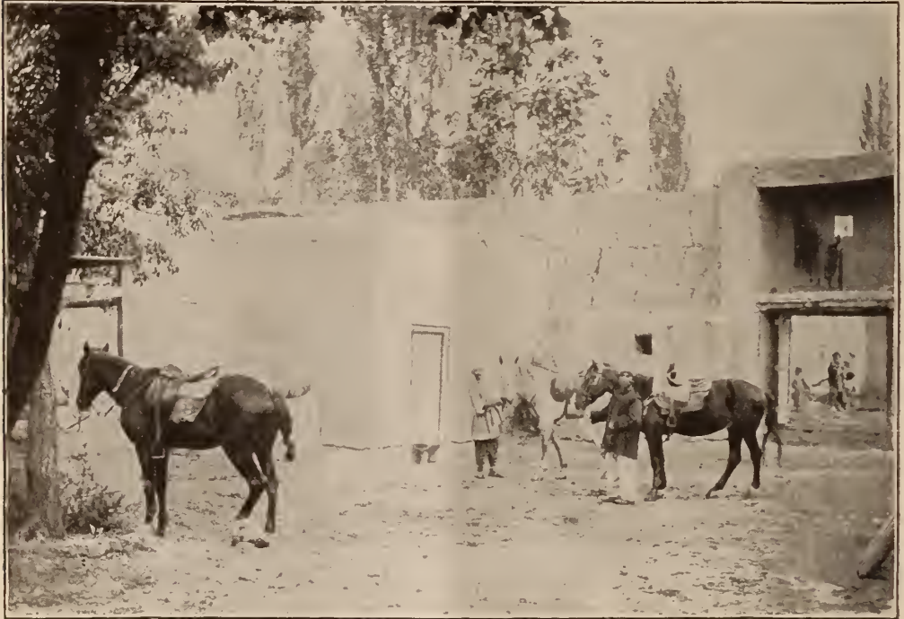
Courtyard, cook-house, street gate and watchman's lodge over the gate of the girls' school at Haft Dewan, Salmas. The house itself is on the right side of the gate and does not appear. It is rented.
